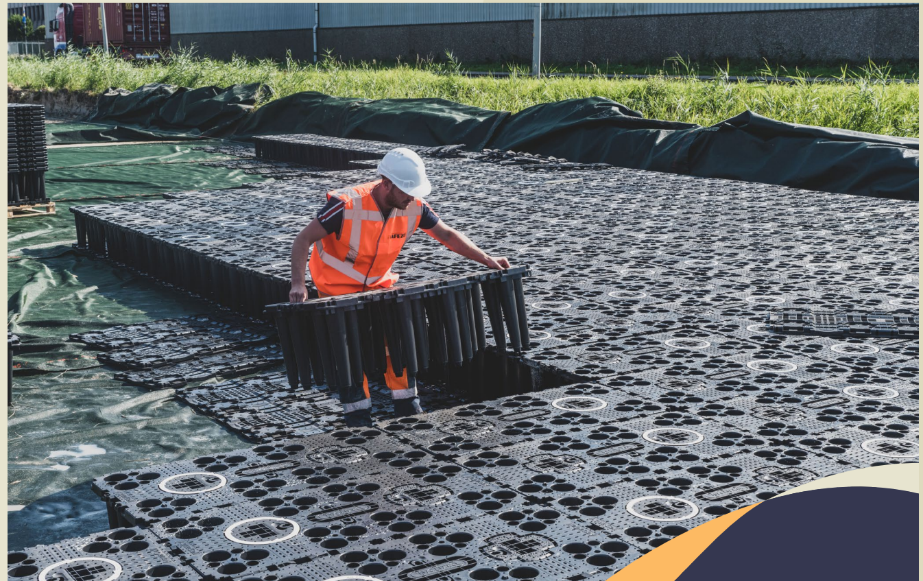
AquaCell infiltration tank made from 100% recycled material
