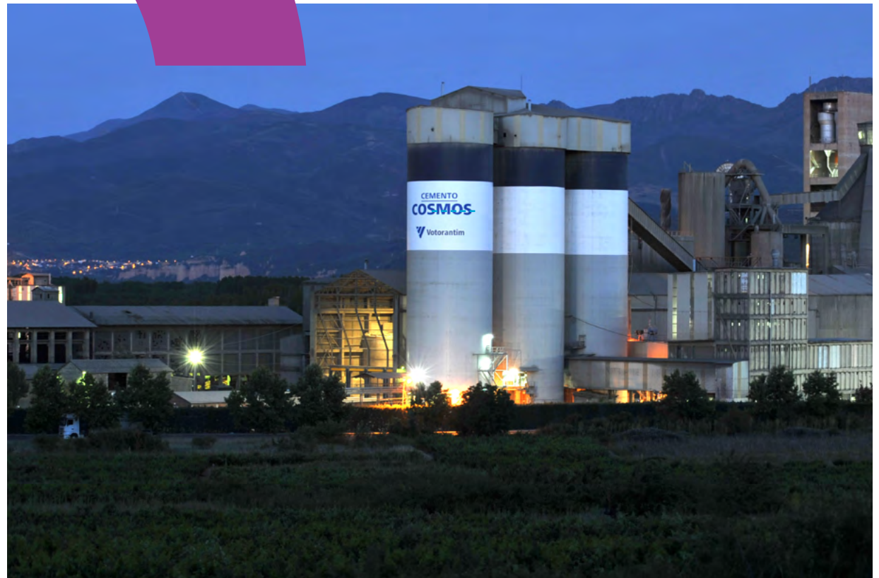
Our plant in Spain that is implementing a solar energy project
