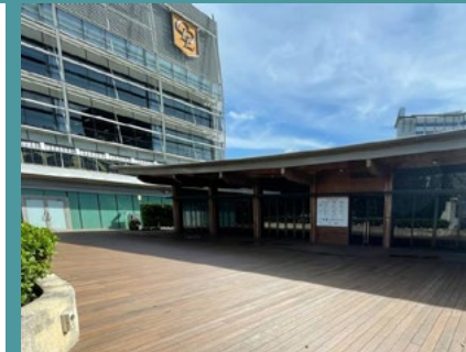
☒ Retrofitted SSA outdoor deck made from 95% recycled materials.
