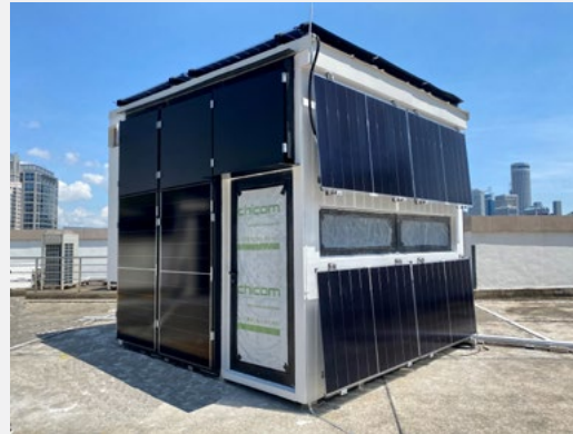
Diagram credit: SERIS, NUS Modular pod installed at Central Mall featuring modular BIPV blocks.
