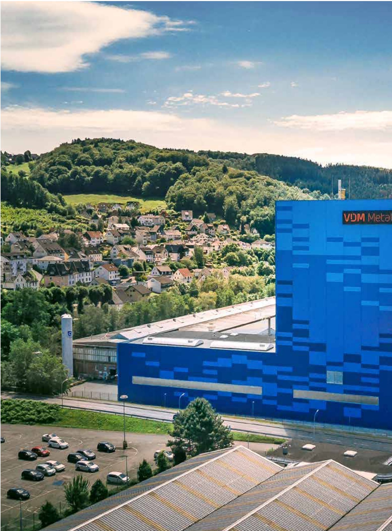
VDM Metals factory in Werdohl (Germany)
