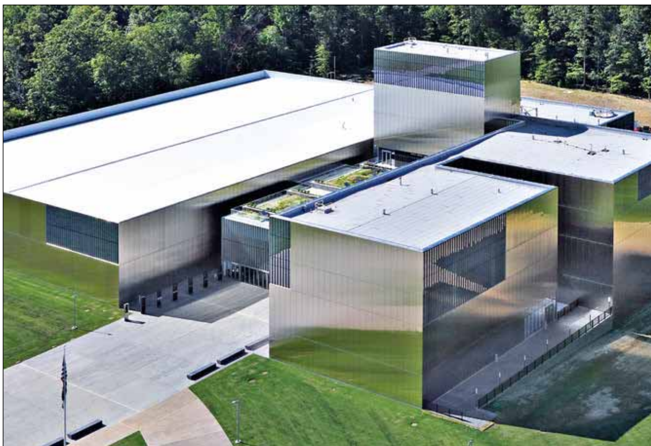
National Museum of the United States Army on the outskirts of Washington D.C., clad with stainless steel sheets supplied by NAS
