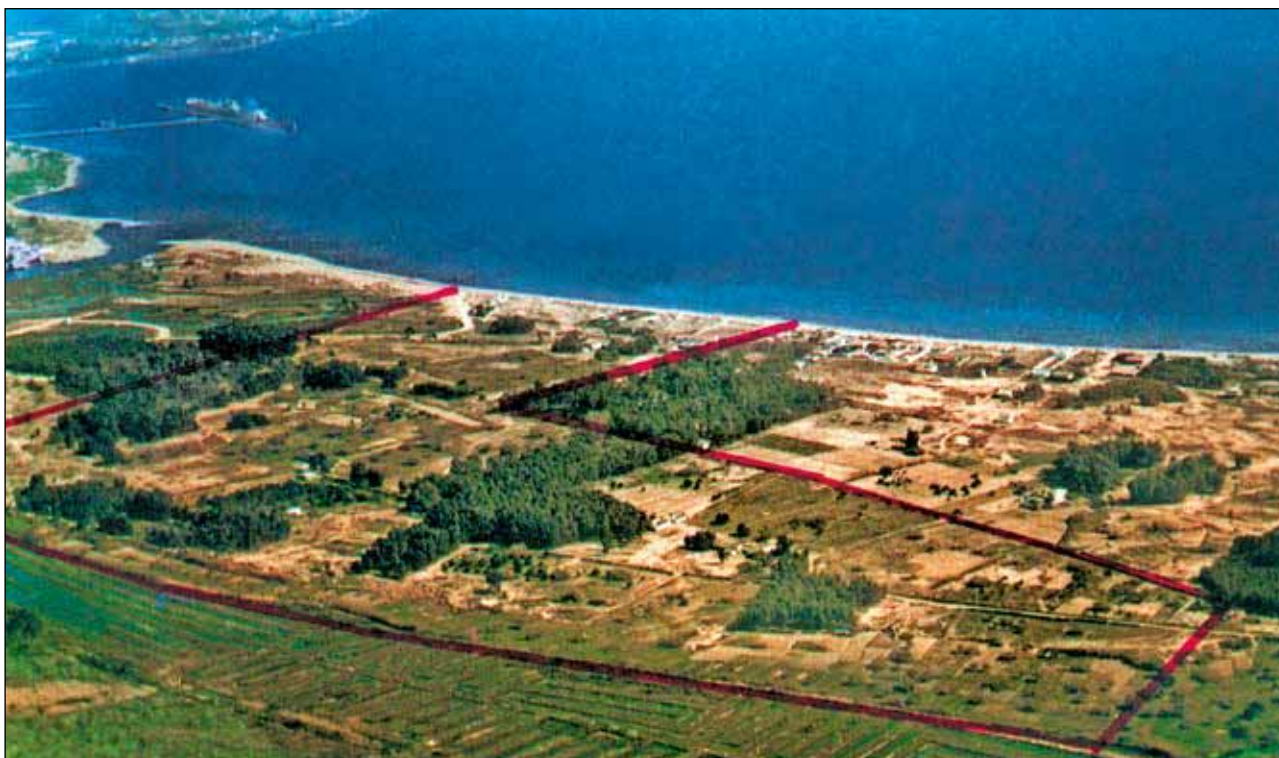
Aerial view of the Acerinox grounds in Campo de Gibraltar (1970)
