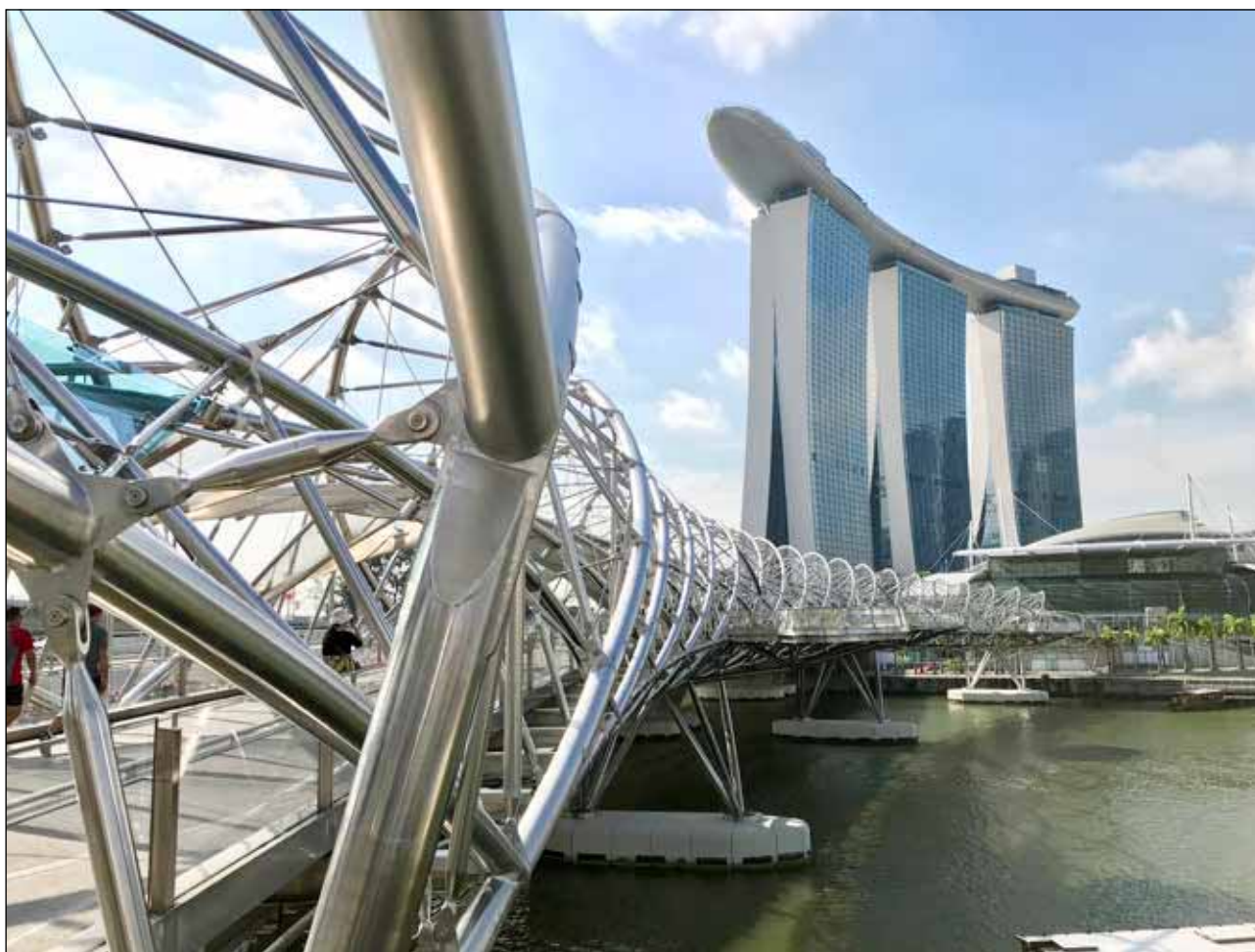
Pedestrian walkway in Singapore
