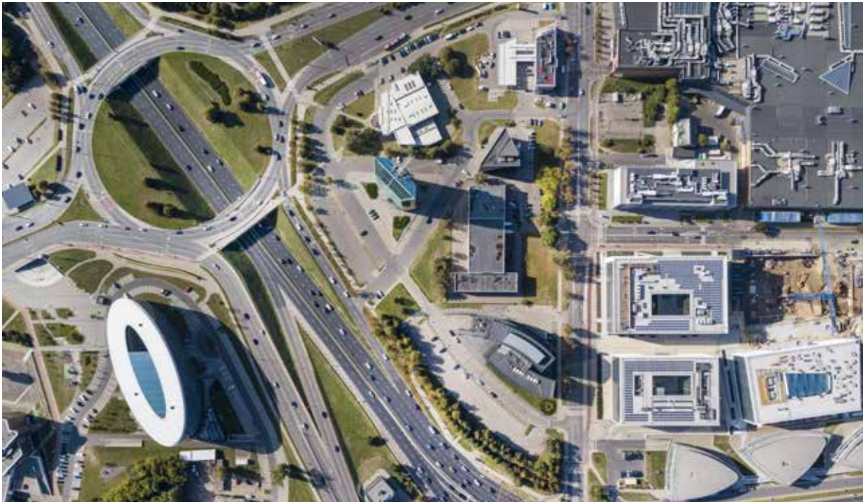
Part of the central business district of Vilnius. At the bottom right of the picture you find Eastnine's S7 properties.
