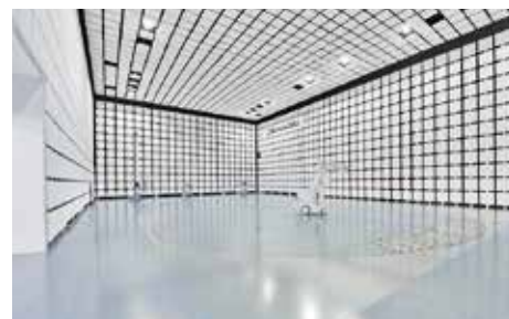
Anechoic Chamber at the Quality Center
