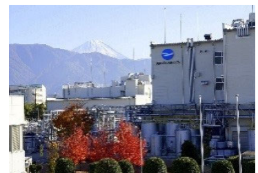
Kofu head office at Konica Minolta Supplies Manufacturing Co., Ltd.
