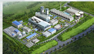
LPG/LNG combined cycle power plant
