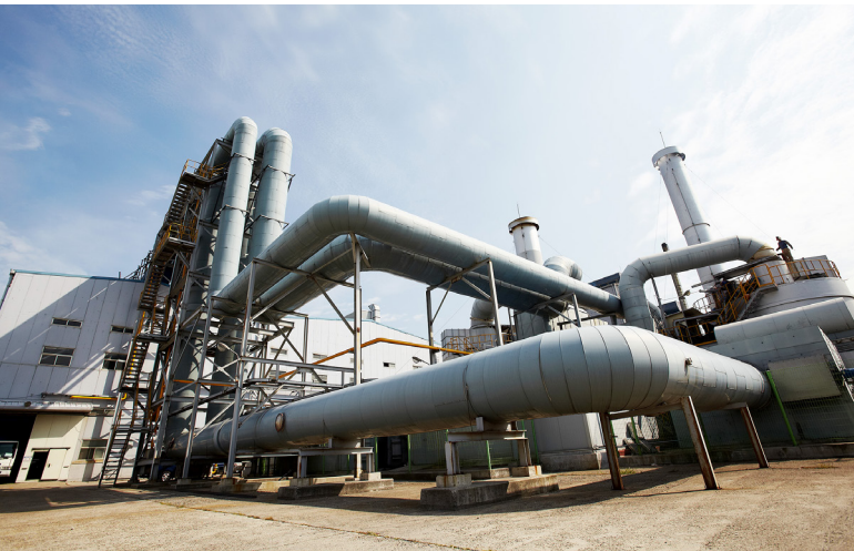
[ Waste Heat Steam Pipes ]
