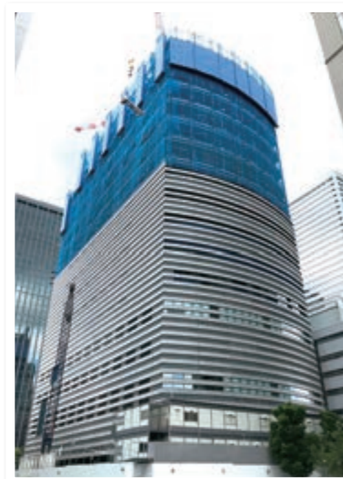
Construction site as of June 2020
