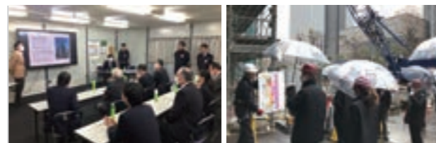
Inspection of the OBP Building construction site by Outside Directors and Audit & Supervisory Board Members
