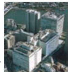
1973 Tokyo Dia Building
