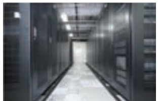
Disaster countermeasure center in the Kansai region
