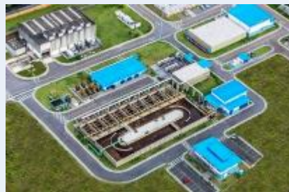
Industrial wastewater treatment plant operated by BRK Ambiental
