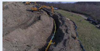
Construction site of a land pipeline
