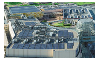
Rooftop solar panels at LaLaport KASHIWANOHA
