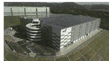
Solar power panels at MFLP Ibaraki (generation capacity approx. 2,000 kW)
