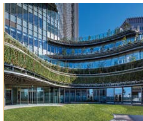
► Wall and roof foliage
