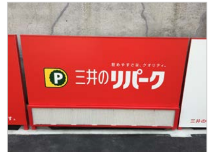
Exhaust gas panel with photocatalytic filter installed at Mitsui Repark's Enkobashi-cho No. 3 Parking Lot in Hiroshima
