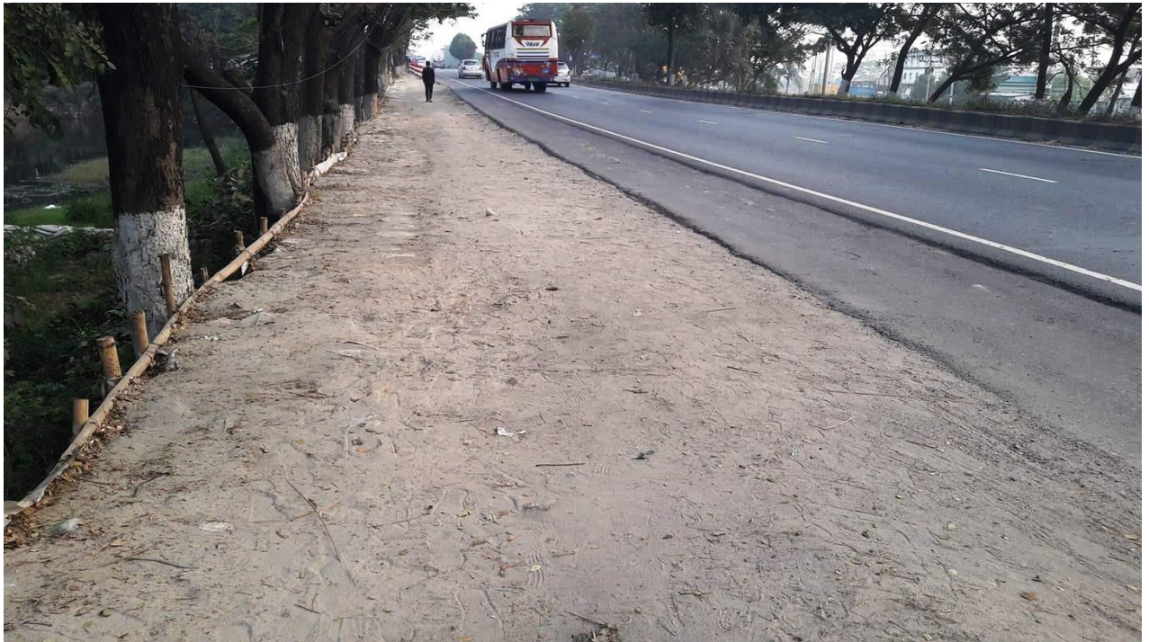
Repaired adjacent road in front of DBPL Factory
