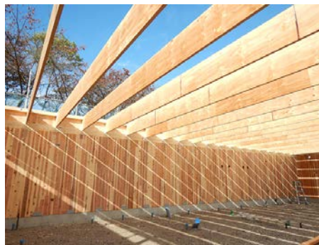
Wood CLT Convenience Store Construction
