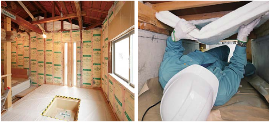
Installation of a Thermal Insulator
