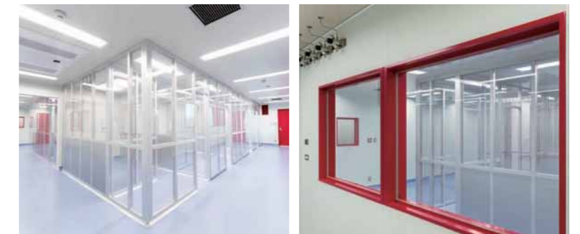
Air Barrier CPF with Air Barrier Booth installed at Cuorips Inc. in July 2020
