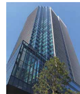
CO-MO-RE YOTSUYA (air conditioning installation)
