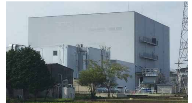
Headquarters Plant, Tokai Capsule Co., Ltd. (air conditioning and plumbing installations)
