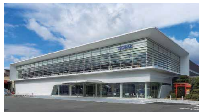
Teral Inc. New ZEB Office (air conditioning and plumbing installations)
