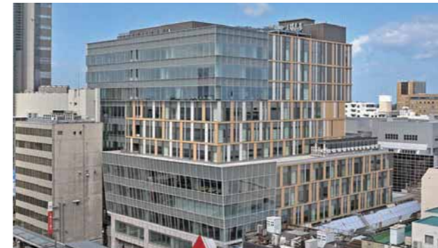
Furumachi Refuru (air conditioning and plumbing installations)
