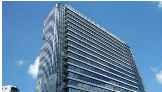
Shibuya Solasta (air conditioning and plumbing installations)
