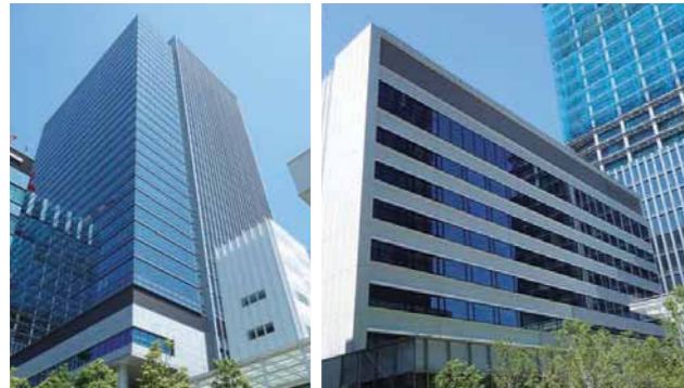
msb Tamachi Station Tower S / Pullman Tokyo Tamachi (air conditioning installation)
