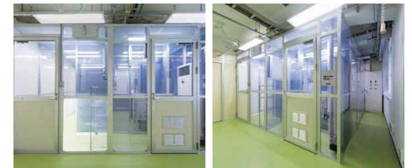
All-in-One CP Unit installed at Mie University in September 2019
