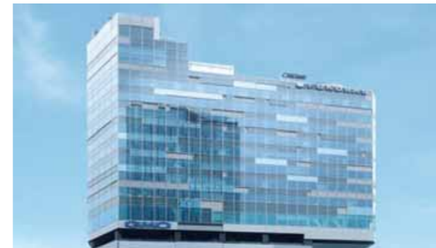
SHIBUYA FUKURAS (air conditioning and plumbing installations)
