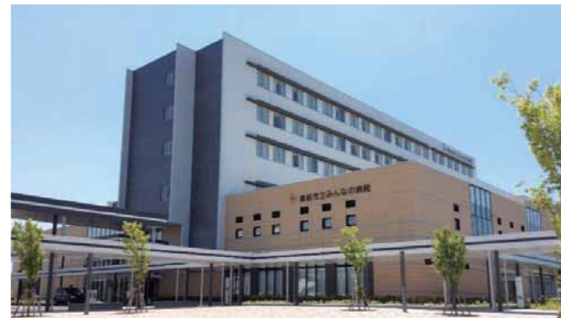
Takamatsu Municipal Hospital (air conditioning and plumbing installations)
