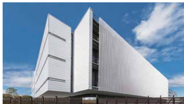
netXDC Sanda Center No. 2 (air conditioning and plumbing installations)
