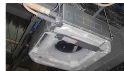
Protects indoor ceiling units against airborne dust and salt during work.
