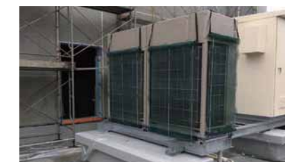
Protects the heat exchanger fins of outdoor AC units against damage caused by inadvertent contact with structures, tools, etc.
