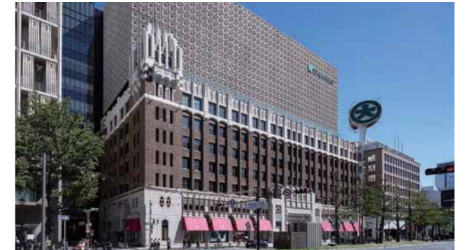
Main Building, Daimaru Shinsaibashi Store (electrical installation)
