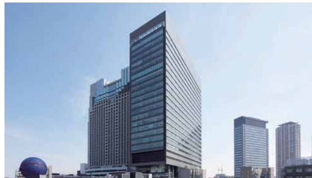
Namba SkyO (electrical, air conditioning and plumbing installations)
