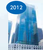
2012 JP Tower, Tokyo
