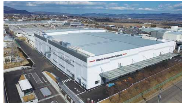
R&D Bldg. and Factory No. 5, Fukushima Plant Hitachi Automotive Systems (air conditioning and plumbing installations)
