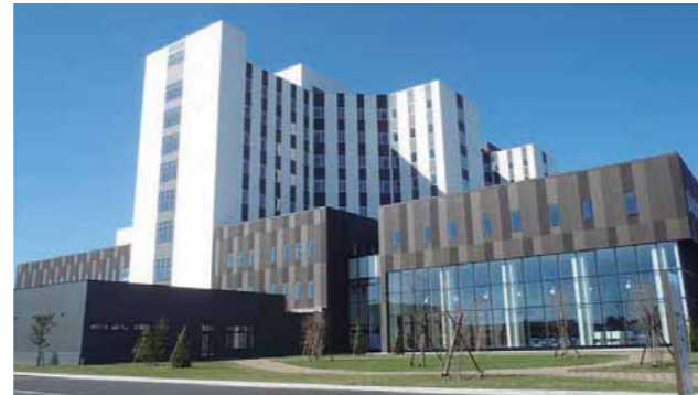
Obihiro Kosei Hospital (plumbing installation)
