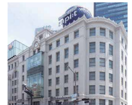
Nankai Terminal Building Nankai Electric Railway Co., Ltd. (electrical installation)
