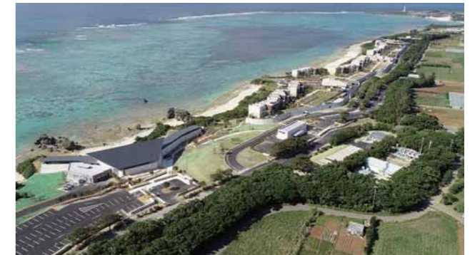
HOSHINOYA Okinawa (air conditioning and plumbing installations)
