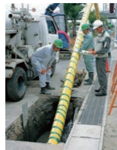
Trenchless pipe installation method
