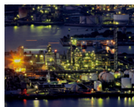
Location: 1-1 Harumi-cho, Shunan-shi, Yamaguchi, Japan Number of employees: 63 Total site area: 70,997m
