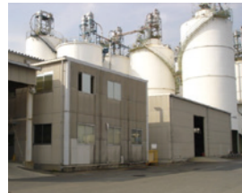
Location: 1-2 Harumi-cho, Shunan-shi, Yamaguchi, Japan Number of employees: 28 Total site area: 3,280m
