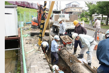
Workers restoring gas service
