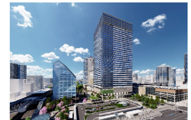
The Toyosu Bayside Cross Tower, which houses the Toyosu Energy Center
