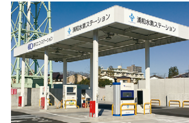
Urawa Hydrogen Station
