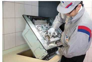
Installing an appliance
