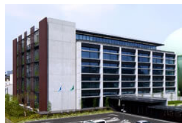
TG Hiranuma Building
