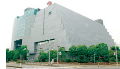
Makuhari District Heating and Cooling Center
