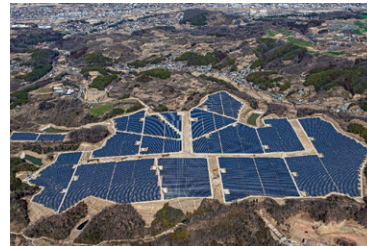
Annaka Solar Power Plant, one of the largest-capacity PV plants in the Kanto Region.
