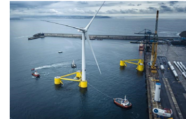
Artist's impression of floating foundation system for offshore wind power plants (Photo provided by Principle Power)
