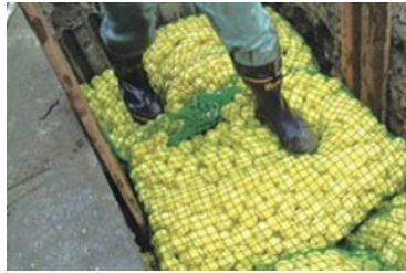
"Eco-balls," an innovative temporary backfiller in pipeline works
