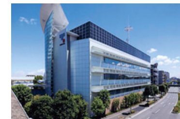
Earth Port (after refurbishment)
