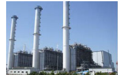
Ohgishima Power Station
