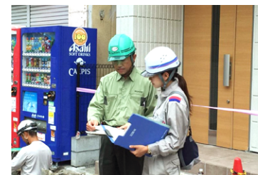
Female employee working at a pipeline construction site.
