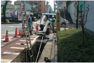
Departure shaft in a non-open cut gas pipeline construction
