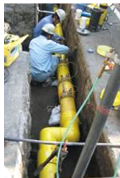
Replacing an aging gas pipe
