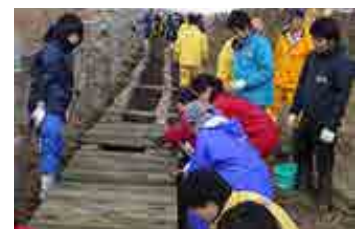
Landscape repair of boardwalk (2014)
