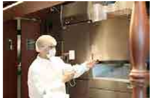
Inspection of kitchen equipment
