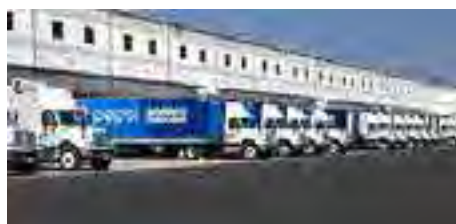
Delivery trucks staged at distribution facility in St. Pauls, North Carolina
