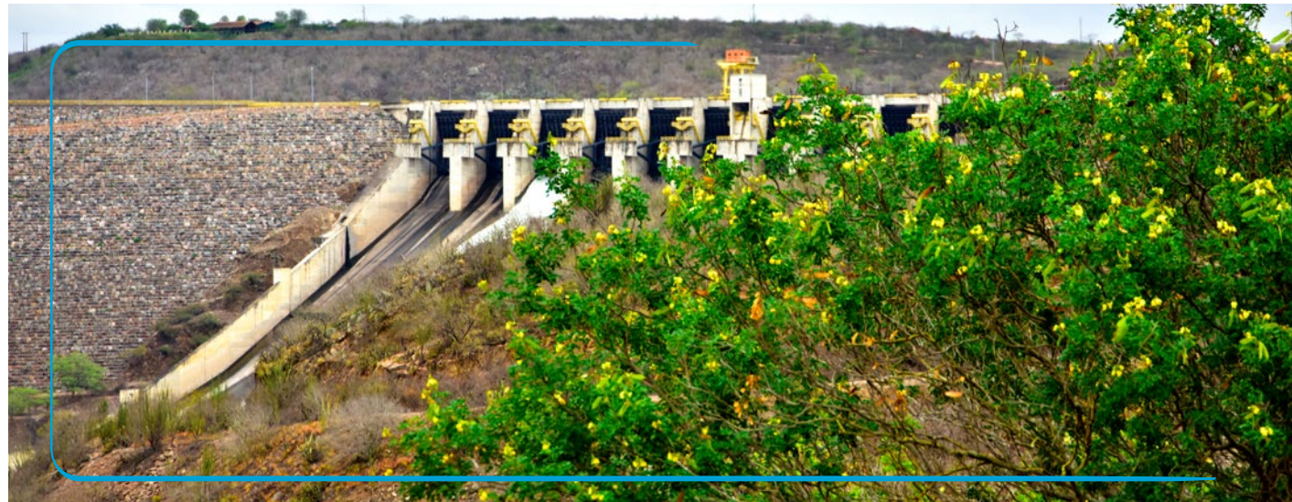
Xingó Hydroelectric Power Plant visitor center, Sergipe. Credit: André Schuler.
