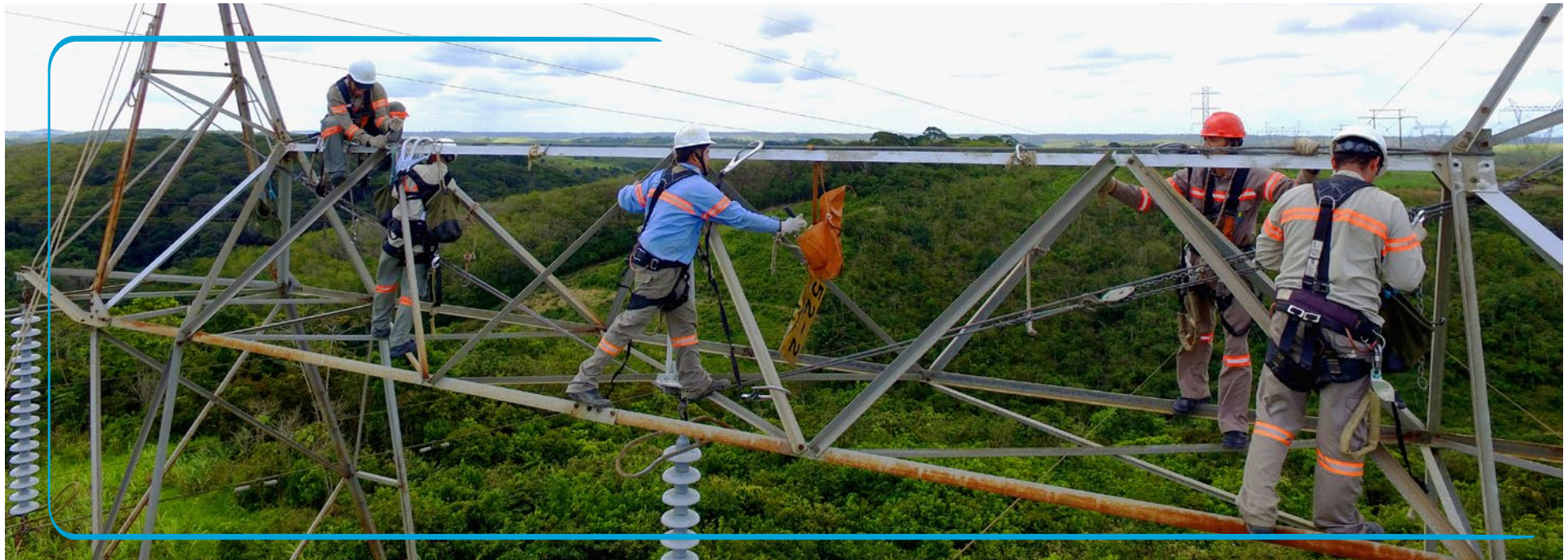
Maintenance on transmission lines. Credit: Eduardo Vilaça.
