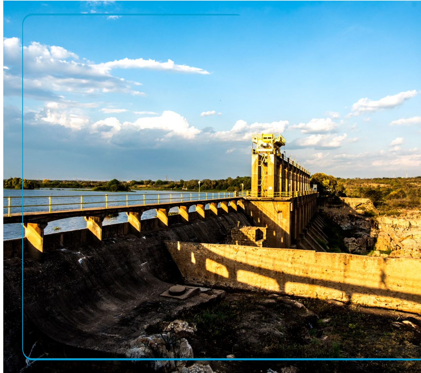
Floodgates of the Paulo Afonso Complex. Photo: André Schuler.
