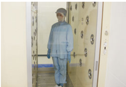
Measures for prevention of contamination by foreign matter (air showers)
