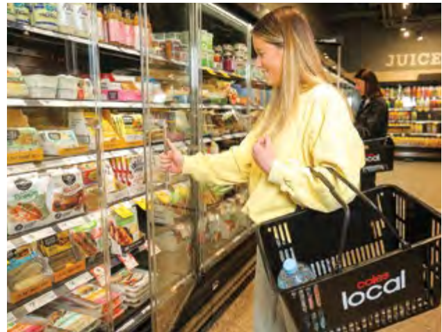
Doors on refrigeration units help to reduce energy consumption.
