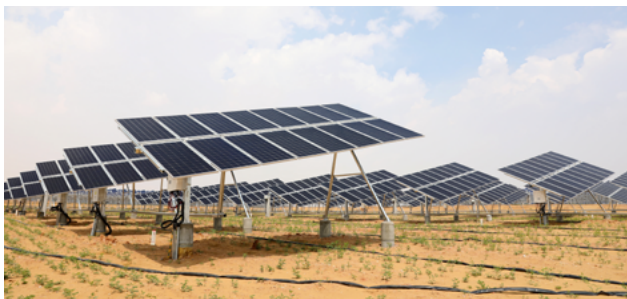
LONGi module products for Kubuqi desertification control project with PV
