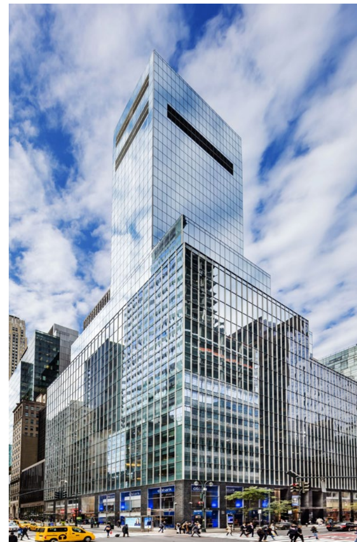
Munich Re Group has agreed to acquire the 330 Madison Avenue building in New York City, designed by Ely Jacques Kahn, LEED Gold certified.
