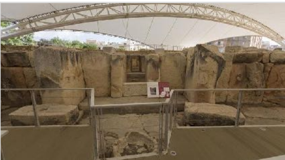
Photo 3: ERDF 32 Archaeological Conservation Project. Cover over the Tarxien Temples 2016. 33
