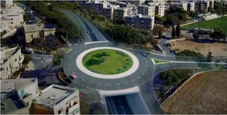
Photo 2: New Santa Lucija Junction currently under tender. 21
