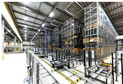
Kyushu Factory and Logistics Center
