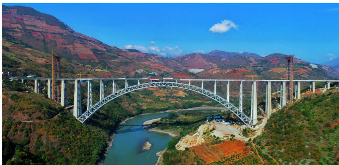
▼ 怒江特大桥 Nujiang Railway Bridge
