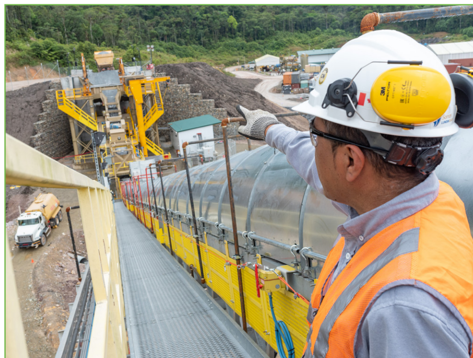
Primary Crusher, Process Plant.
