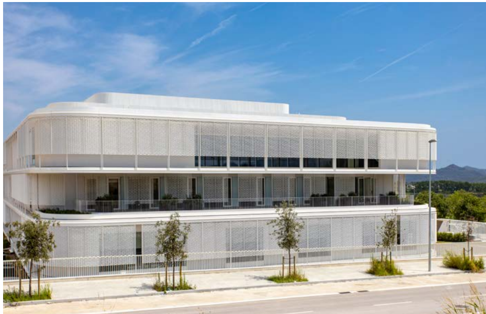
New Natura Bissé corporate headquarters, Cerdanyola del Vallès (Spain)
