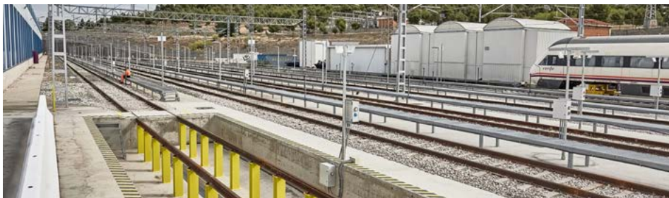
Rail yard expansion of high-speed train at the base of Santa Catalina, Madrid (Spain)
