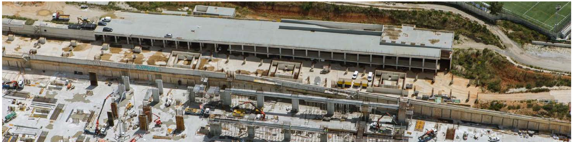
Construction of the AVE station in La Sagrera, Barcelona (Spain)
