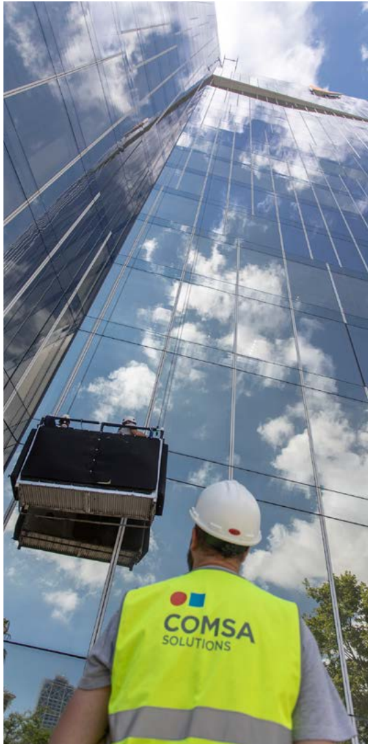
Cleaning work carried out by COMSA Solutions
