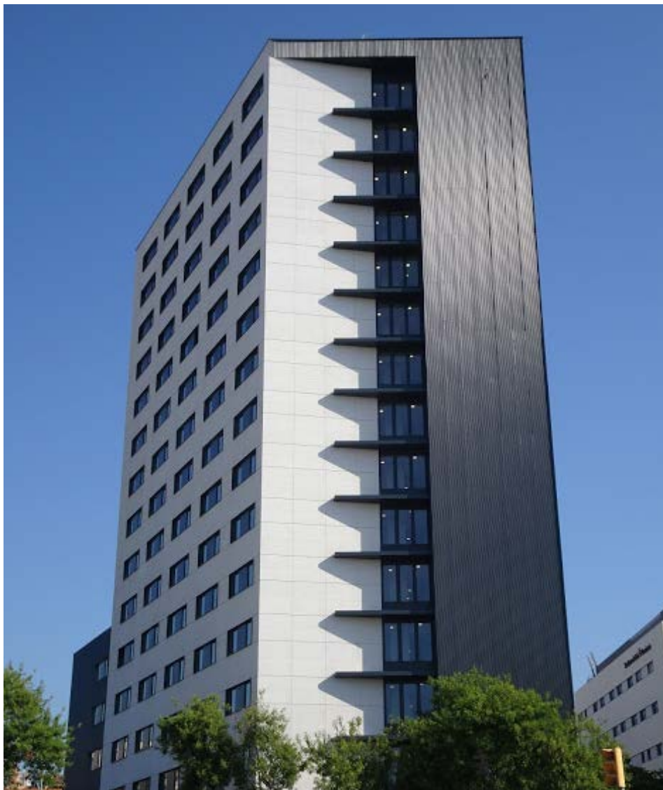
Construction of a Student Residence near Sants Station, Barcelona (Spain)
