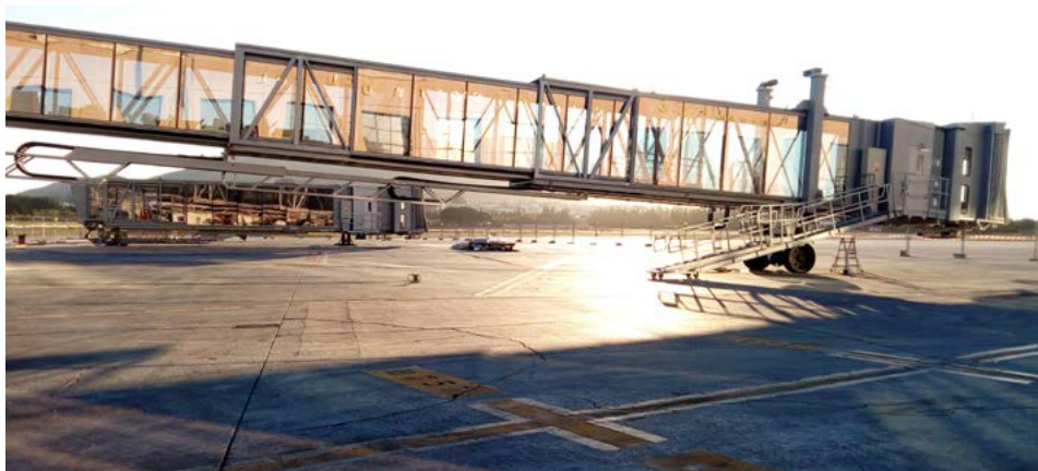
Installation of boarding bridges and auxiliary equipment, Malaga airport (Spain)
