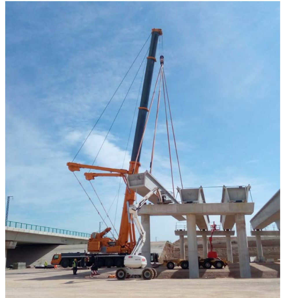
Construction of the Reguerón Highway, Murcia (Spain)
