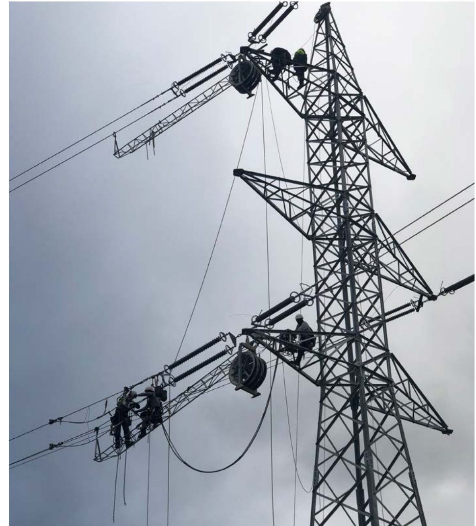
Substations and associated transmission lines of four ENEL Green Power Iberia wind farms (Spain)
