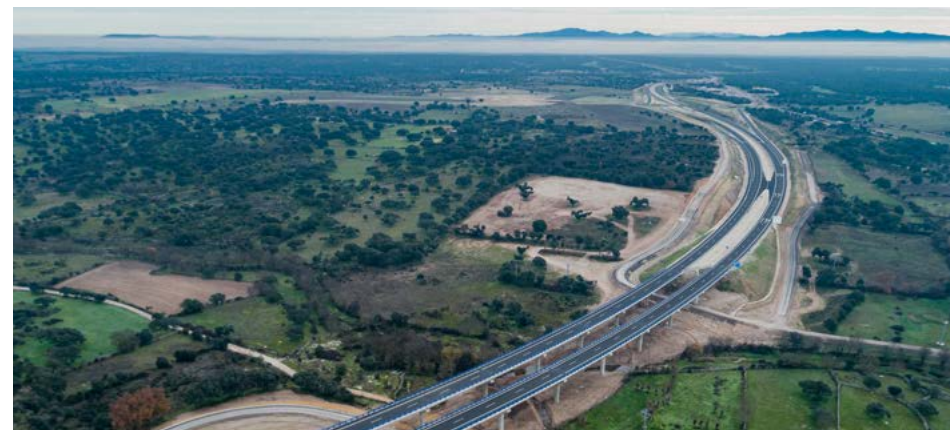
Castilla A-62 motorway. Section: Fuentes de Oñoro, Border between Portugal and Salamanca (Spain)
