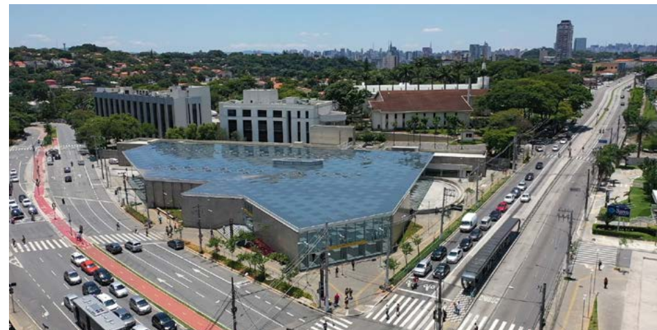
Second phase of Metro Line 4, Sao Paulo (Brazil)
