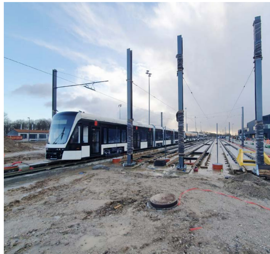
Tram section under construction, Odense Tram (Denmark)
