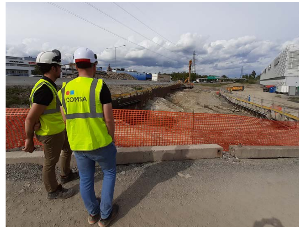
Construction of two access tunnels to the E4 motorway, Stockholm (Sweden)
