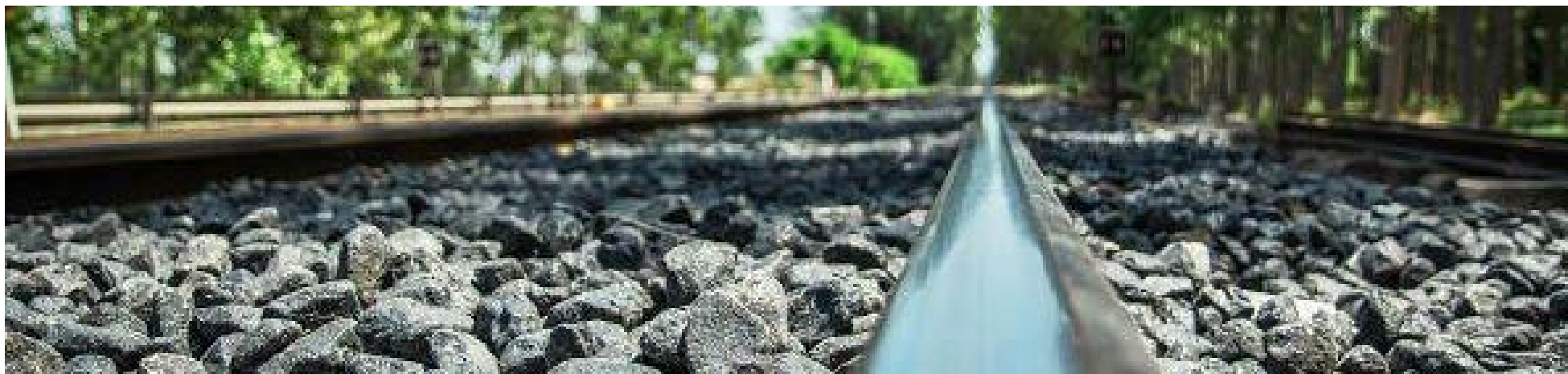
Neoballast field test section between Maçanet-Massanes and Caldes de Malavella section, Girona (Spain)
