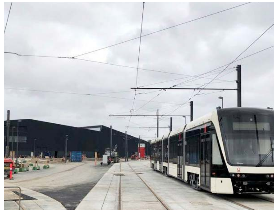
Tram construction, Odense (Denmark)
