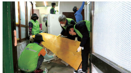
Supporting Renovation of Old housing
