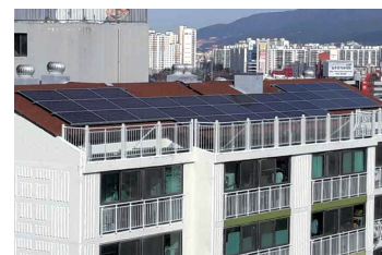
Installing Solar Power Facilities for Rental Housing
