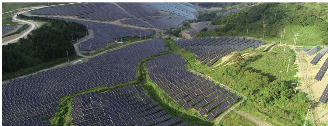
Green loans (Solar power plant facilities)
