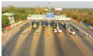
Sagaing Highway 188 km of toll road connecting 3 major cities in Upper Myanmar
