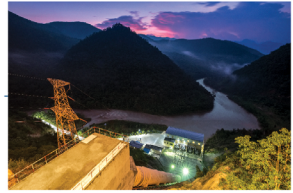
Baluchaung 3 52 MW hydropower plant powering the country
