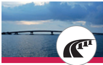
BRIDGES AND FLYOVERS
