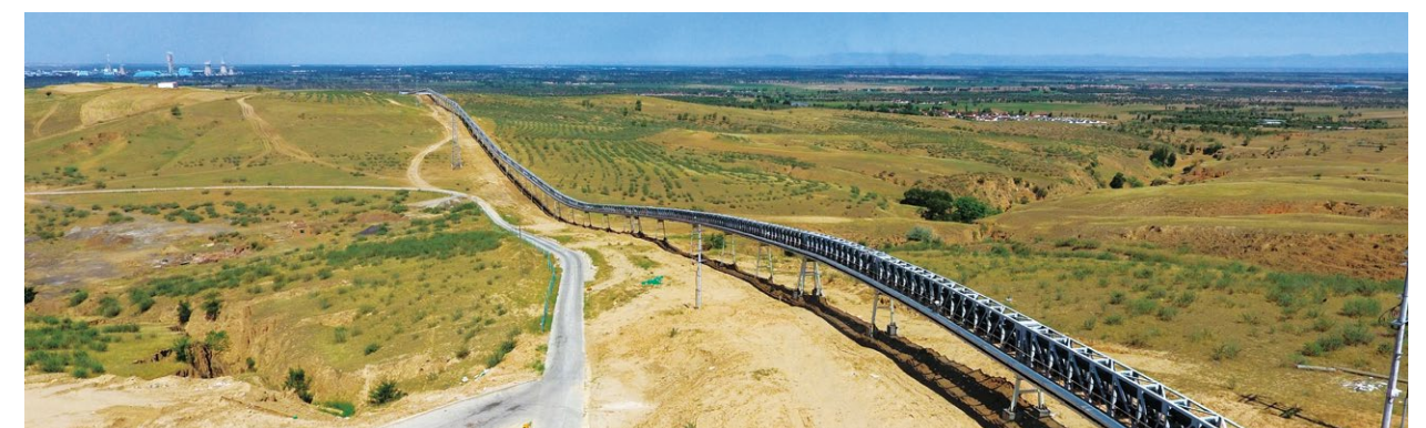
▲ The Kulyuetu Ditch Watershed Comprehensive Governance Project of Inner Mongolia Tuoketuo Power Plant
