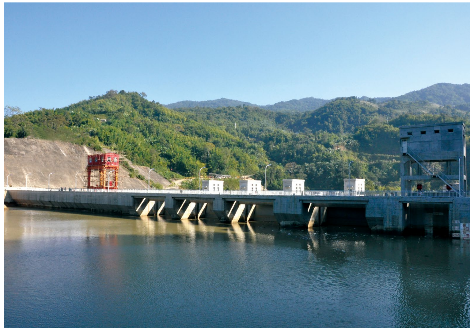
▲ The Taipingjiang River Hydropower Plant in Myanmar runs safely and steadily, and ensures local power supply. In 2019, its power generation volume reached 920 GWh.
