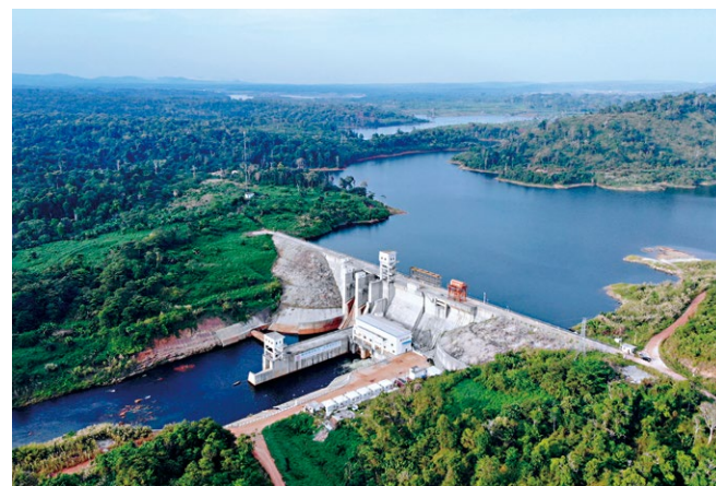
▲ The Stung Atay Hydropower Project in Cambodia runs safely and steadily, and delivers favorable benefits. In 2019, its power generation volume reached 186 GWh.
