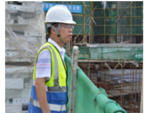
Checking equipment working aloft
