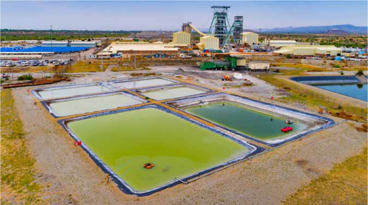
Styldrift Mine with storm water and settling dams in the foreground
