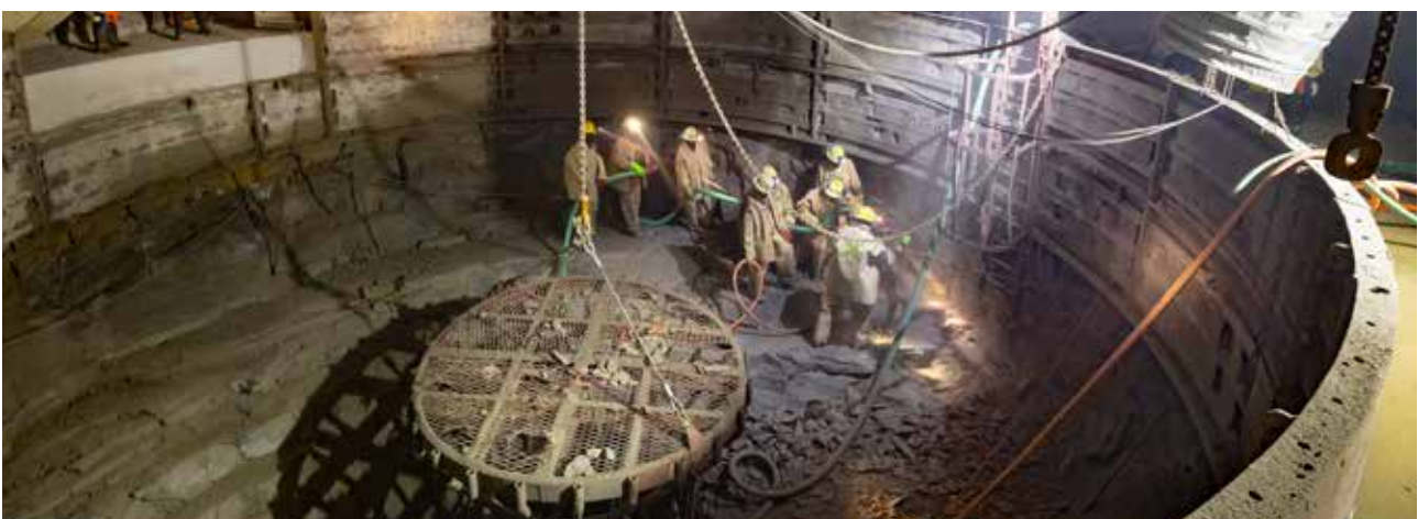
Styldrift Settler No 2 collar construction
