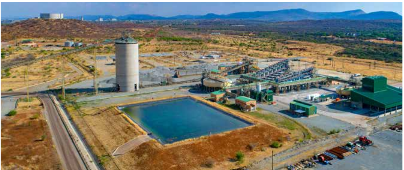
Aerial view of Maseve concentrator and mill feed silo
