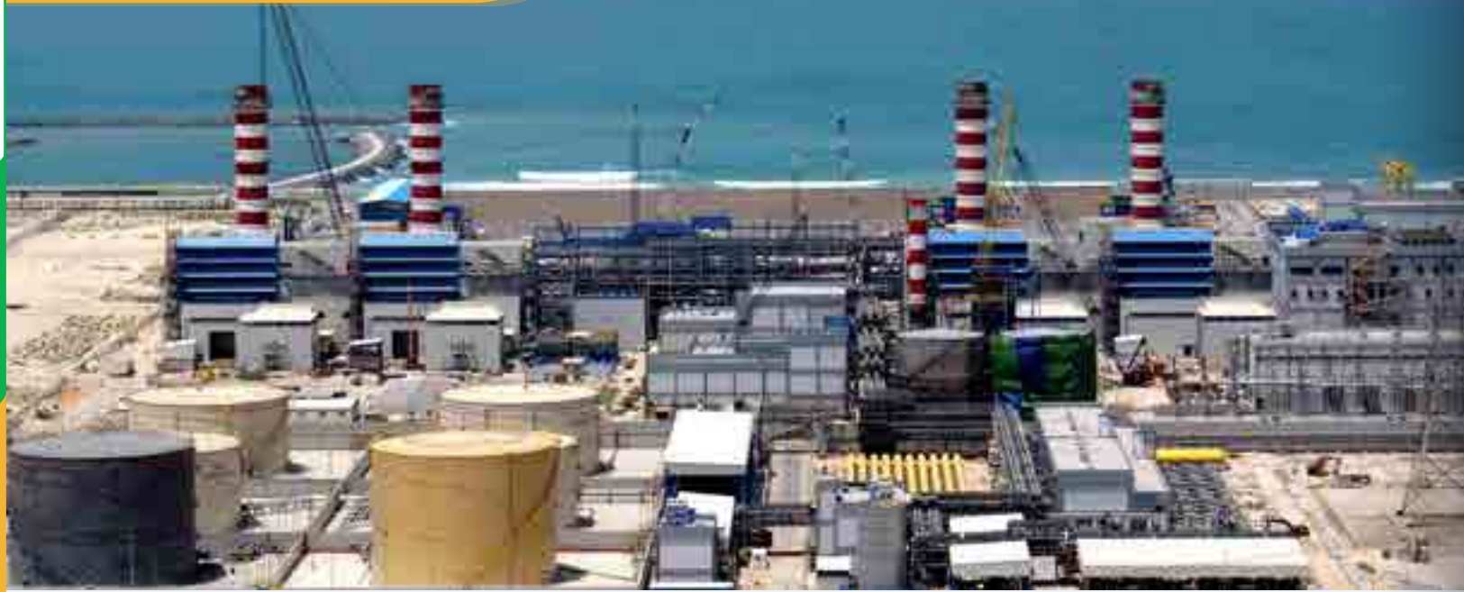
Jebel Ali Power and Water Desalination Complex
