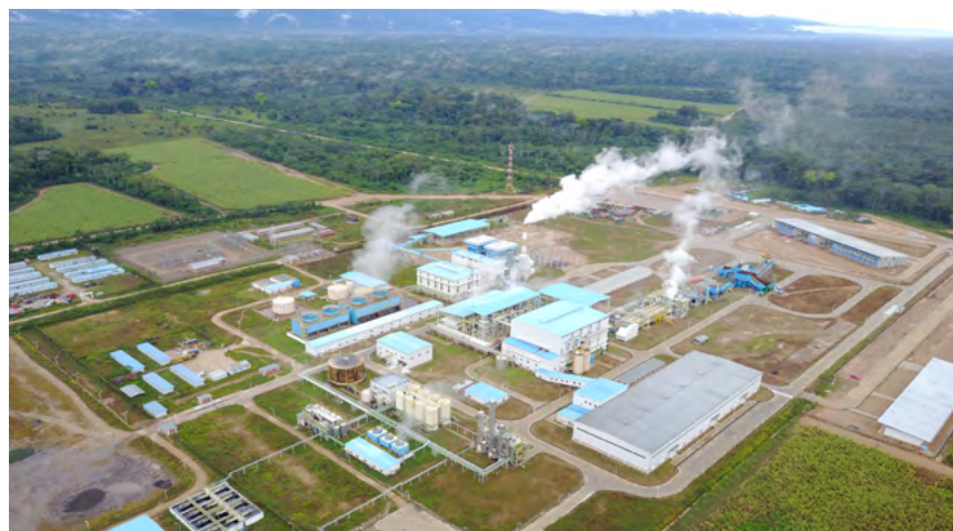
◆ The San Buenaventura sugar factory project in Bolivia constructed by CAMCE
