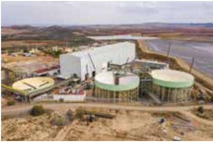
Pyrites plant construction at Fresnillo
