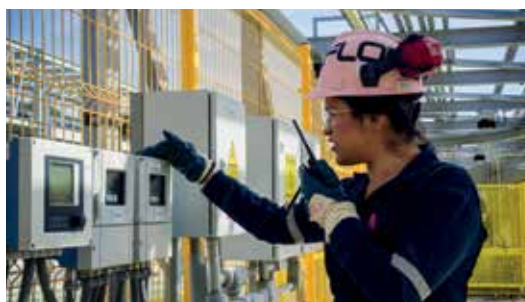
An employee at the Merrill Crowe plant at San Julián
