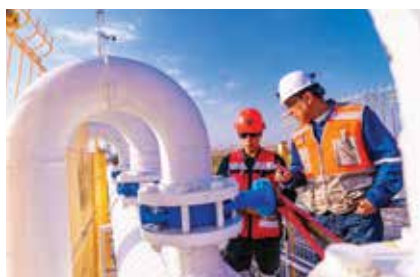
Water treatment plant in the Fresnillo district
