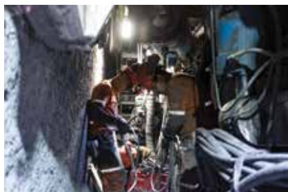
Engineers working at the tunnel boring machine at Fresnillo
