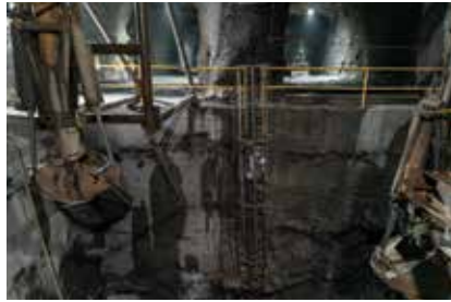
Deepening of the San Carlos shaft at Fresnillo
