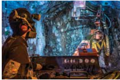
A jumbo drill at work underground
