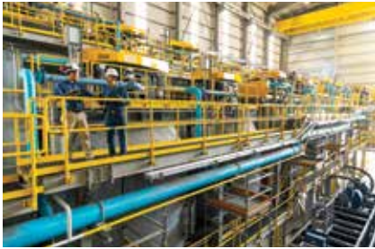
The expansion of the flotation plant at Fresnillo
