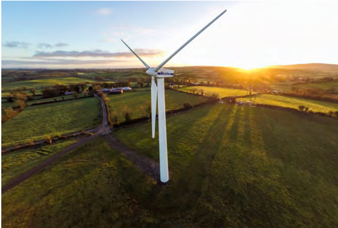
Figure 30 - NTR Bann Energy's Refurbished Bonus 300 turbine at Trillick, Northern Ireland
