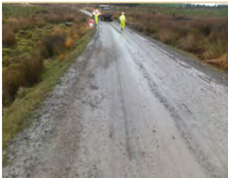
Figure 47 - A wheel loss ‘near miss’ incident at Castlecraig Wind Farm
