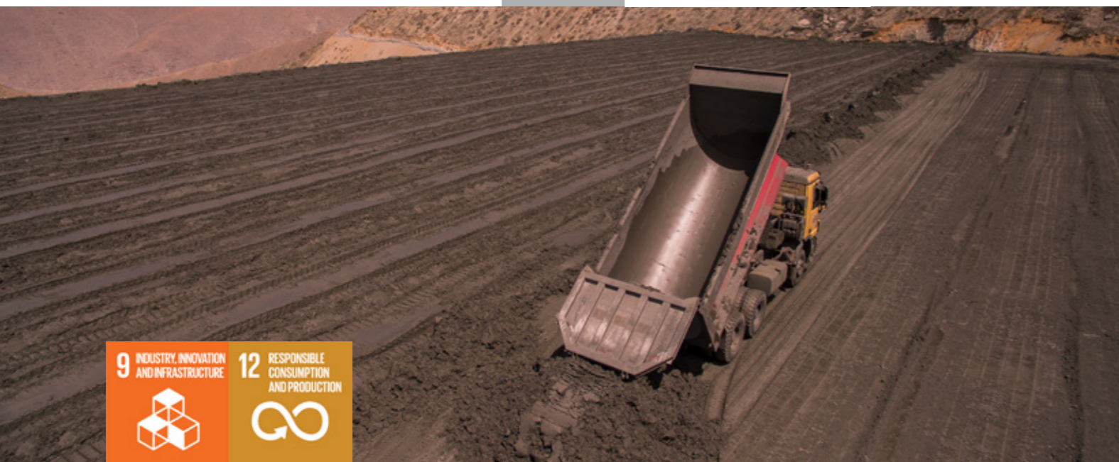
Dry stacking in Cerro Lindo
