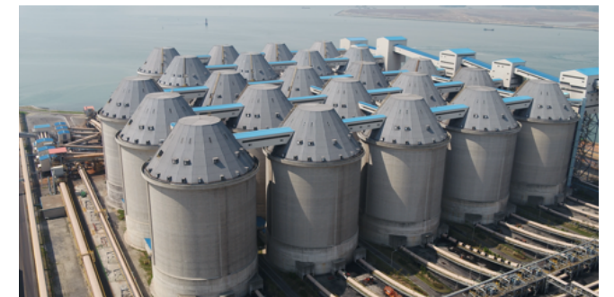
Fully-enclosed fuel/raw material silo at the Gwangyang Works
