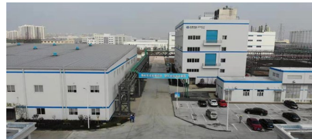
Cathode plant in Zhejiang, China
