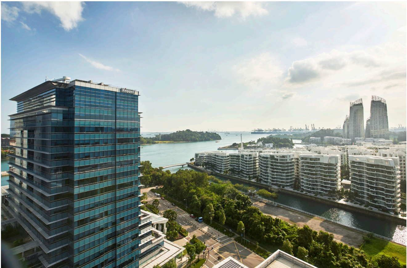
As a leading green developer, Keppel Land develops sustainable and innovative live-work-play environments of enduring value. Testament to the Company's efforts, Keppel Bay Tower (in foreground), located in the world-class Keppel Bay waterfront precinct, is on track to become Singapore's first super low-energy high-rise existing commercial building. The BCA Green Mark Platinum development is also fully powered by renewable energy.
