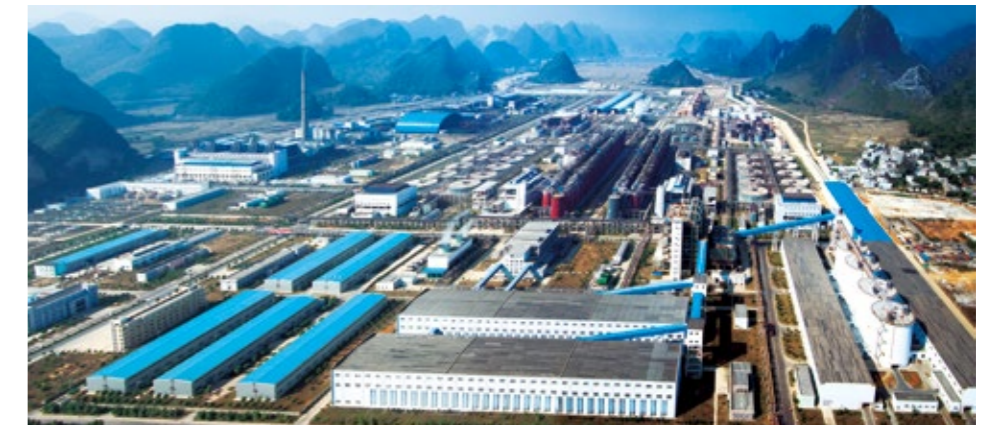
The plant of Guangxi Huayin Aluminium Co., Ltd.
