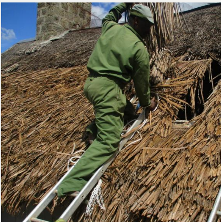
Replacing Makuti (coconut leaf roofing)
