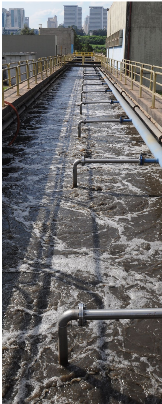
Tank of the Company's largest sewage treatment plant, ETE Barueri, in the west of Greater São Paulo
