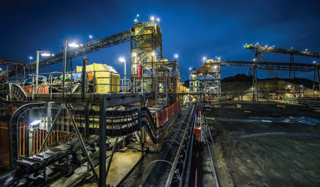
Karowe Mine processing plant
