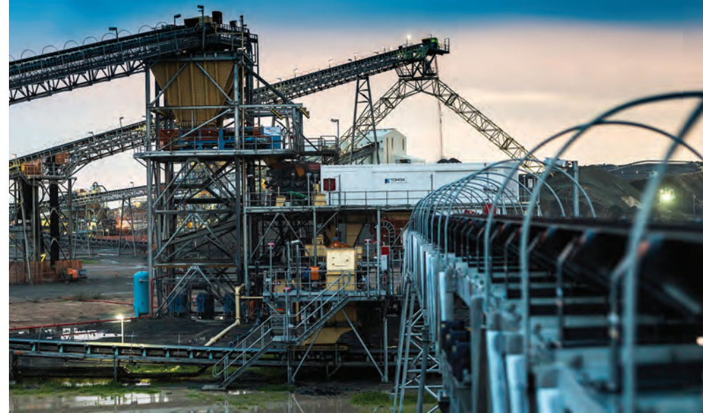
Karowe processing facility
