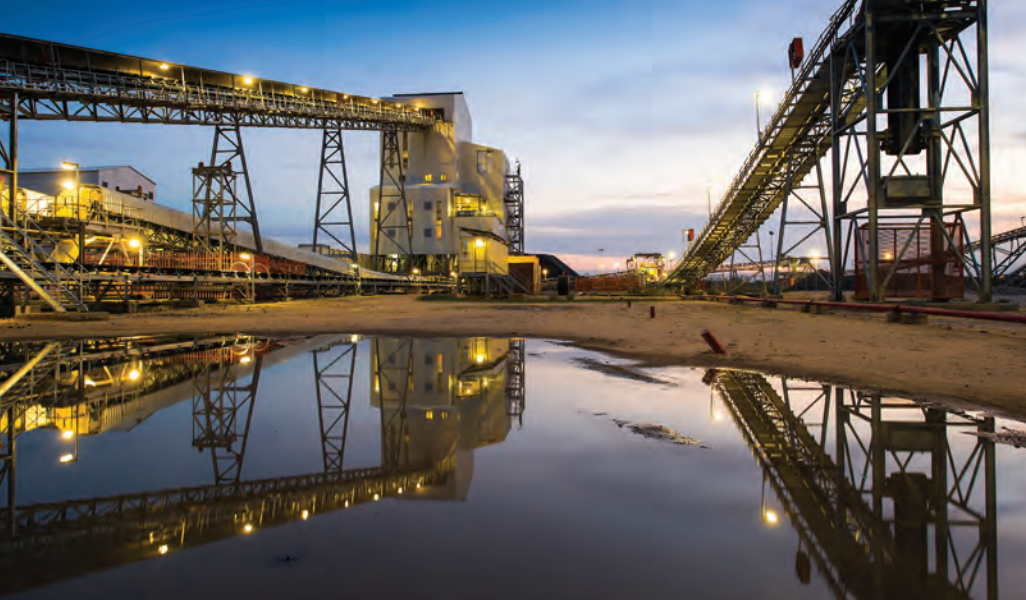
View of conveyors and processing plants at Karowe
