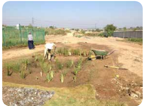
Figure 15: Planting of one of the swales in process.
