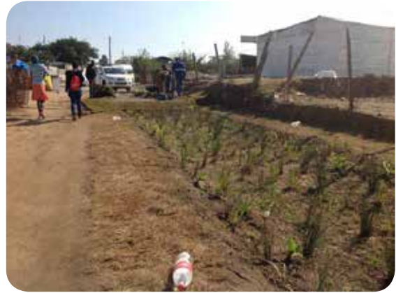
Figure 20: Swale on the Ward 095 site after a three-day long rain event.
