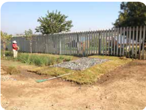
Figure 19: Grass planting around the reno mattress and sedimentation for erosion protection.
