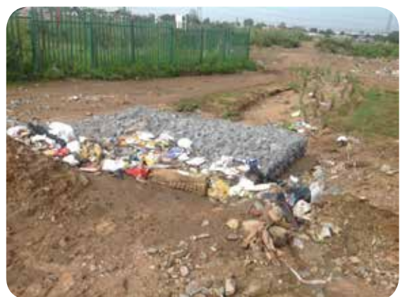
Figure 16: Reno mattress placement on top of sedimentation tank completed; soil levels still need to be completed.
