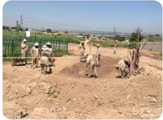
Figure 14: Community workers levelling the swale profile before planting.
