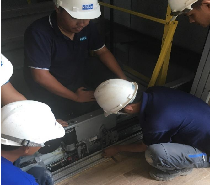
KONE- LIFT DOOR ADJUSTMENT TRAINING
